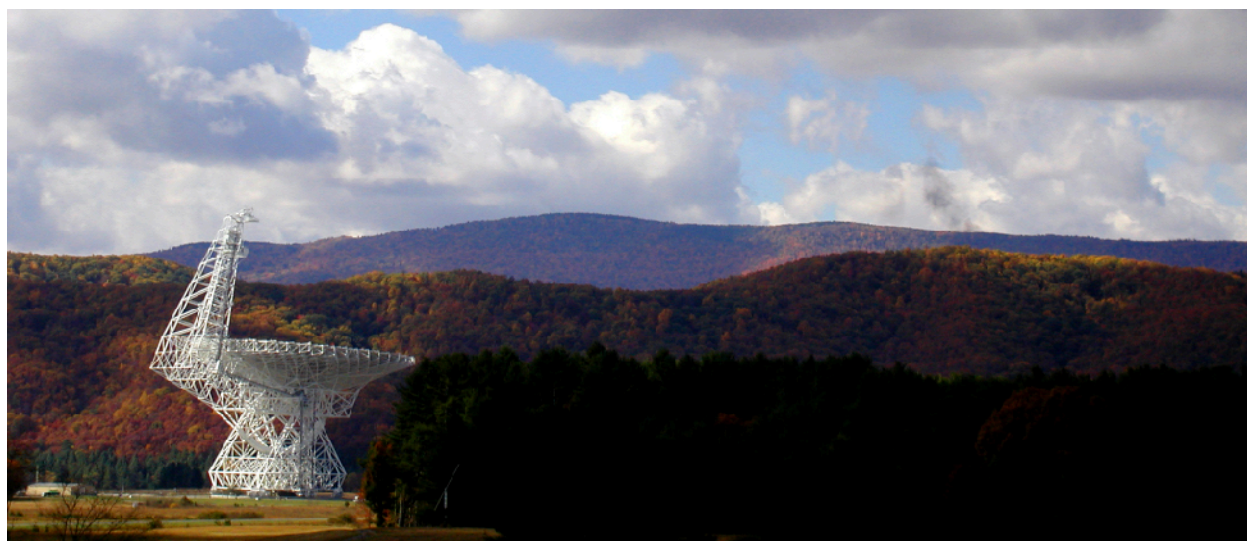
Figure 34.19 This fully steerable radio telescope in West Virginia went into operation in August 2000. Its dish is about 100 meters across. (credit: modification of work by “b3nscott”/Flickr)
