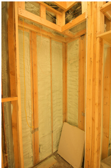
Figure 16.20 Insulation is used to limit the conduction of heat from the inside to the outside (in winter) and from the outside to the inside (in summer). (credit: Giles Douglas)
