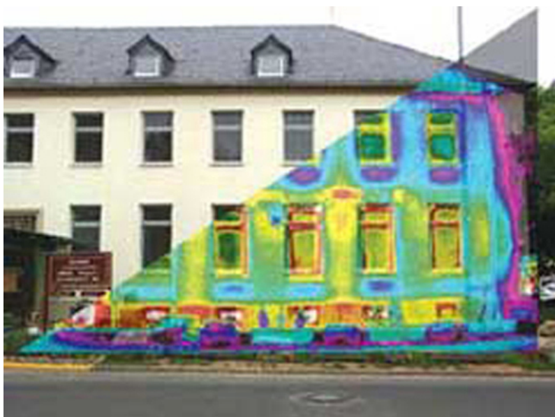
Figure 16.32 A thermograph of part of a building shows temperature variations, indicating where heat transfer to the outside is most severe. Windows are a major region of heat transfer to the outside of homes. (credit: US Army)
