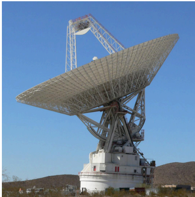
Figure 23.3 This dish-shaped antenna, part of the NASA Deep Space Network in California's Mojave Desert, is 70 meters wide. Nicknamed the "Mars antenna," this radar telescope can send and receive radar waves, and thus measure the distances to planets, satellites, and asteroids. (credit: NASA/JPL-Caltech)
