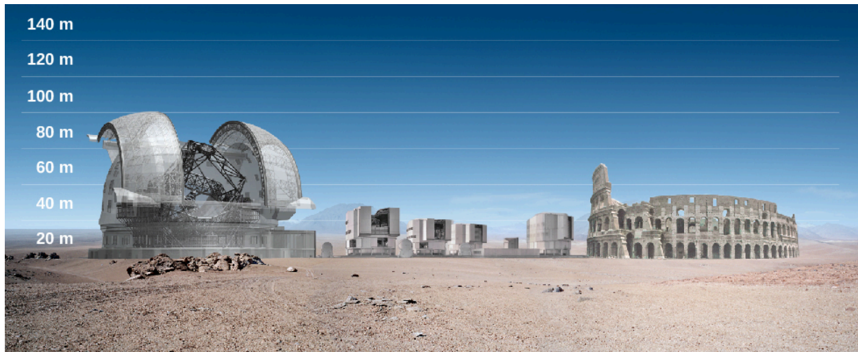
Figure 29.6 The European Extremely Large Telescope (E-ELT) is currently under construction in Chile. This image compares the size of the E-ELT (left) with the four 8-meter telescopes of the European Very Large Telescope (center) and with the Colosseum in Rome (right). The mirror of the E-ELT will be 39 meters in diameter. Astronomers are building a new generation of giant telescopes in order to observe very distant galaxies and understand what they were like when they were newly formed and the universe was young. (credit: modification of work by ESO)
