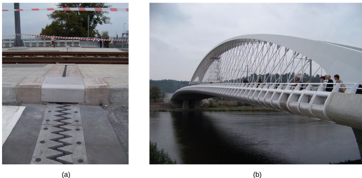
Figure 16.5 (a) Thermal expansion joints like these in the (b) Auckland Harbour Bridge in New Zealand allow bridges to change length without buckling. (credit: modification of works by “ŠJů”/Wikimedia Commons)
