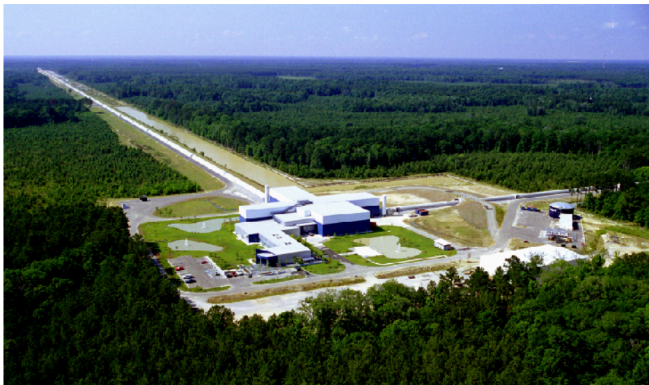
Figure 25.31 An aerial view of the LIGO facility at Livingston, Louisiana. Extending to the upper left and far right of the image are the 4-kilometer-long detectors. (credit: modification of work by Caltech/MIT/LIGO Laboratory)
