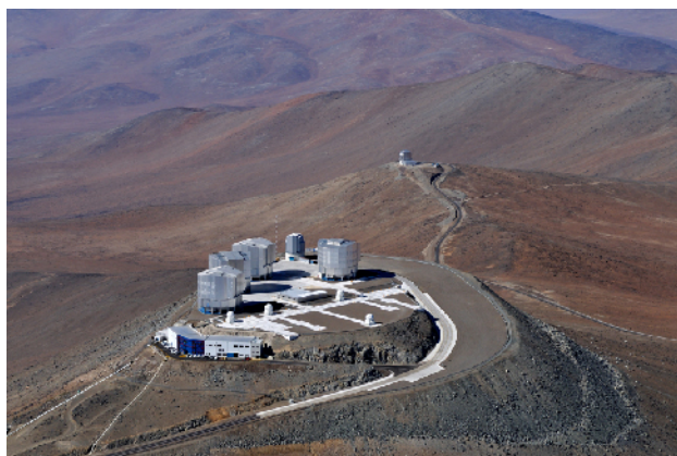
Figure 34.12 Cerro Paranal, a mountain summit 2.7 kilometers above sea level in Chile’s Atacama Desert, is the site of the European Southern Observatory’s Very Large Telescope. This photograph shows the four 8-meter telescope buildings on the site and vividly illustrates that astronomers prefer high, dry sites for their instruments. The 4.1-meter Visible and Infrared Survey Telescope for Astronomy (VISTA) can be seen in the distance on the next mountain peak. (credit: ESO)
