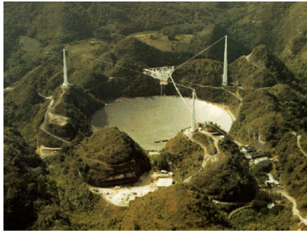
Figure 34.22 The Arecibo Observatory, with its 1000-foot radio dish-filling valley in Puerto Rico, is part of the National Astronomy and Ionosphere Center, operated by SRI International, USRA, and UMET under a cooperative agreement with the National Science Foundation. (credit: National Astronomy and Ionosphere Center, Cornell U., NSF)
